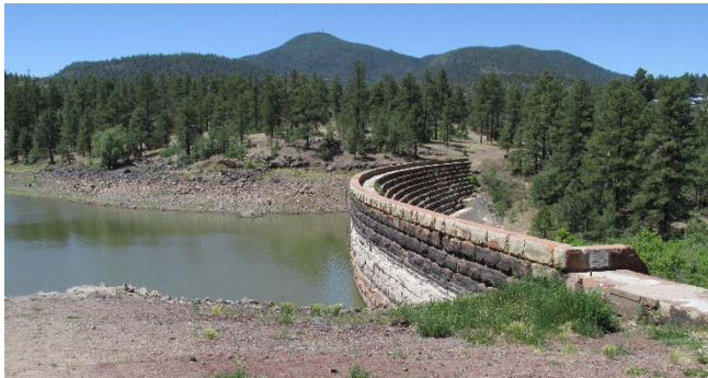
City of Williams Santa Fe Reservoir
